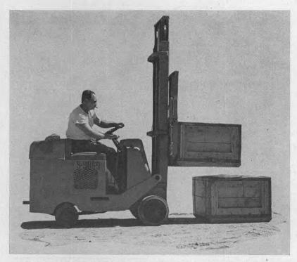
THE HANDIEST GADGET on the base is the fork lift. They come in all sizes and shapes from little box lifters to monstrous machines that can hoist 18,000 pound crates 20 feet in the air with ease. Raymond Summer, 2124-1, uses a 3,000-pound fork lift here to stack small crates.
